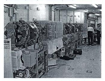
Installation of the magnets in the storage ring. Magnets are colour-coded according to type. The closest (green) is a hexapole magnet, the next closest (red) is a quadrupole magnet, and the large (yellow) magnet is a dipole magnet. Magnets are supplied by CMS Alphatech and Buckley Systems, New Zealand.
